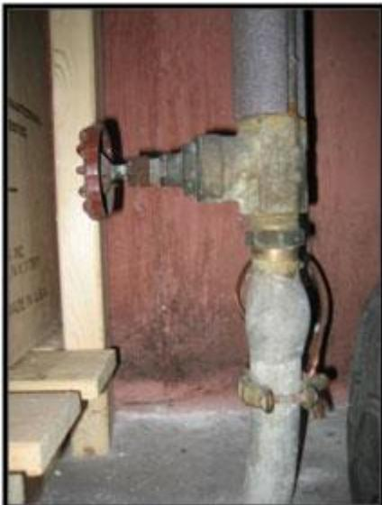
**Pic. 3 (left):** Lead service lines often end just inside the front or side wall of the home, but may extend further into the building.
